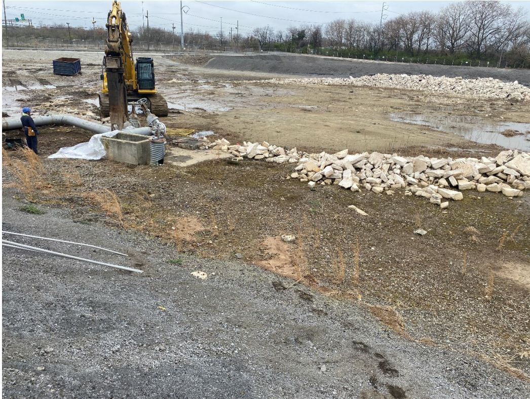
Photographs taken during pipe removal.
