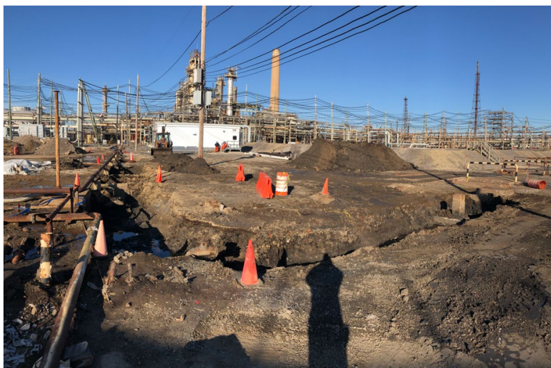
November/December 2019 Excavation Extent (Stantec 2019)
