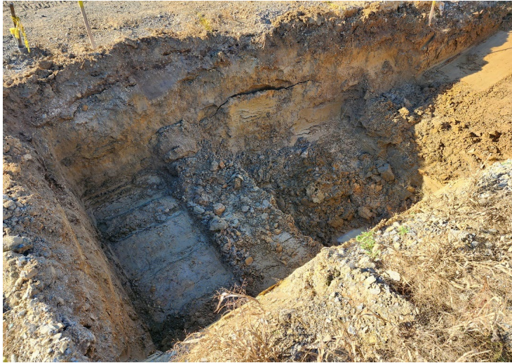
November 2022 Excavation, Area 2 (Ransom)
