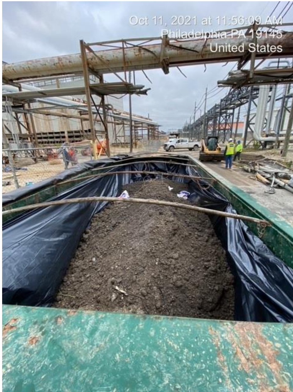
View of sorbent material from roadway and excavated soil in Roll-off
