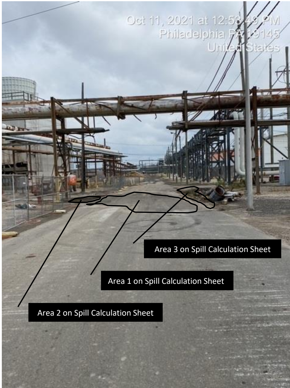
Looking east at release area (Post Cleanup)
