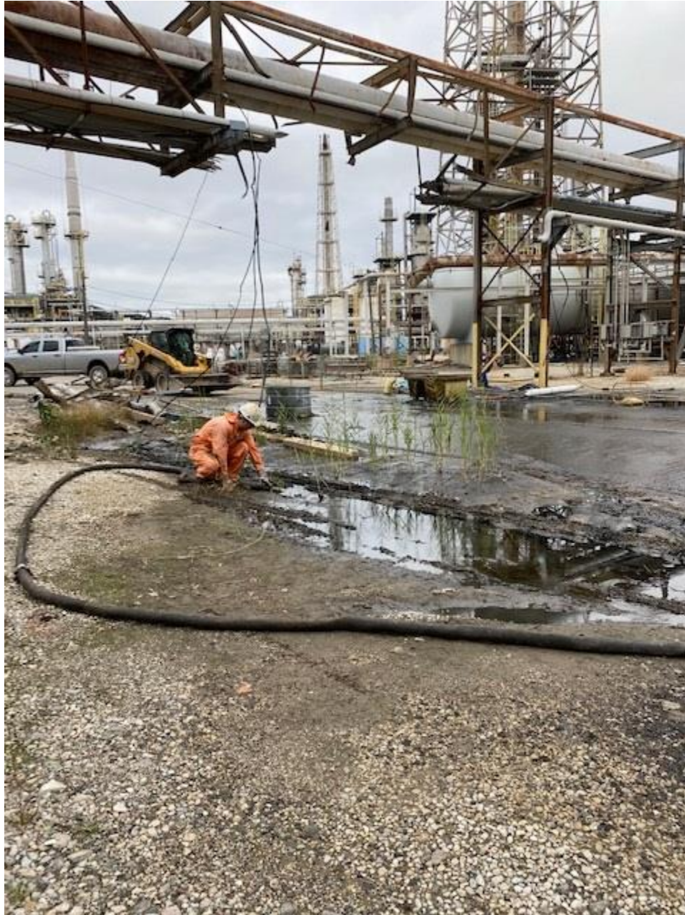
Vacuuming oil and wash water from Area 2 of the spill calculation Sheet. Water was decanted from the vacuum truck (estimated 500 gallons) and remaining oil placed in tank 272 slop oil tank for future sale.
