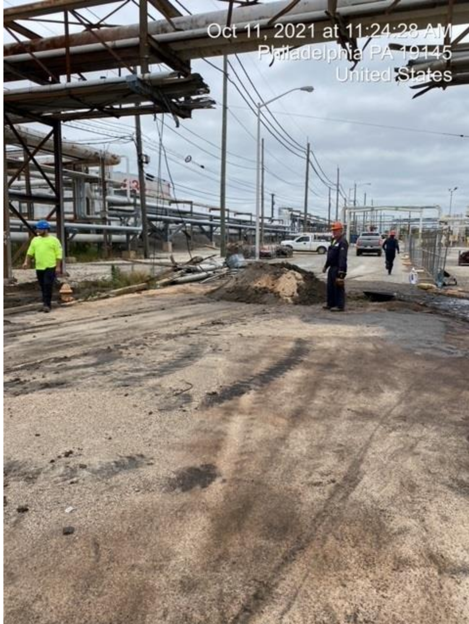
Sorbent material and excavated soil being stockpiled while waiting for a lined roll-off to arrive from the empty container laydown area.
