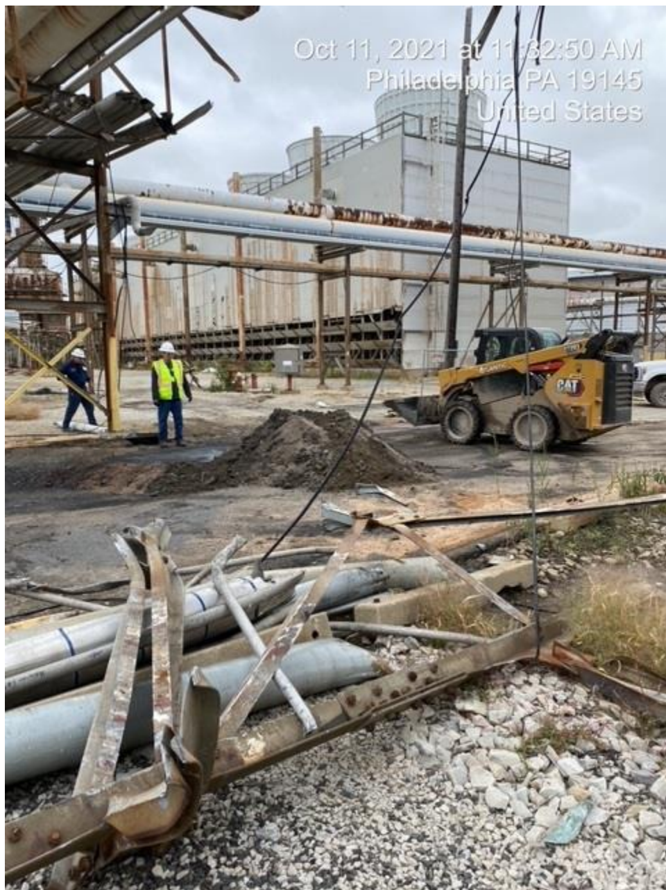
Looking northeast as sorbent material and excavated soil is stockpiled.
