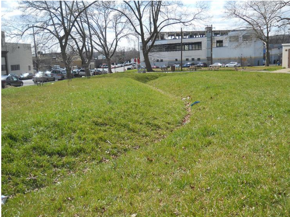
Example from PWD Stormwater Guidance Manual
