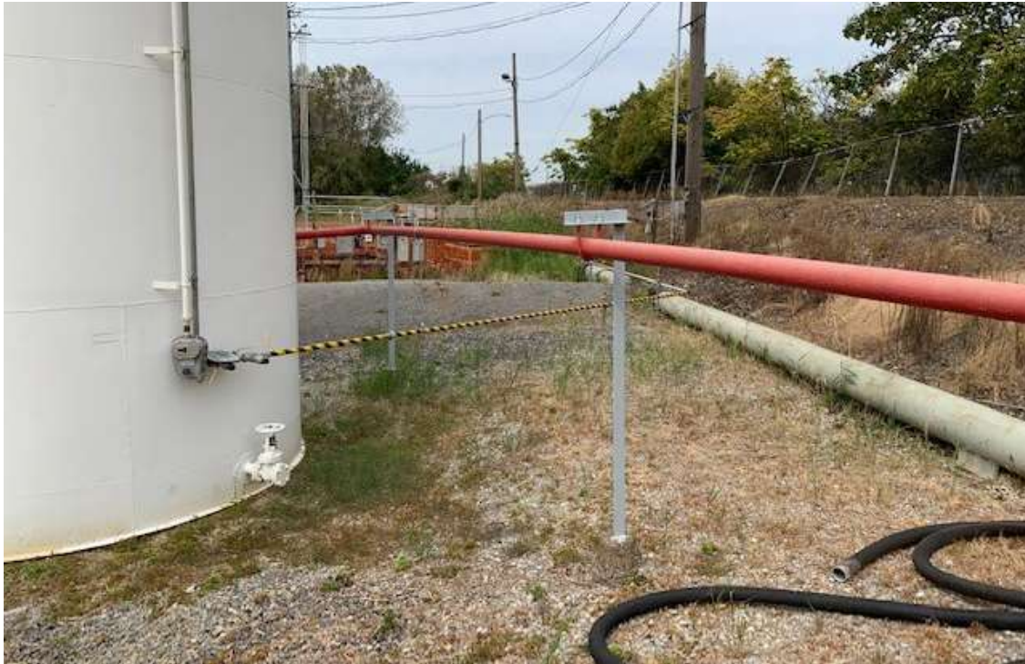
Photo 3: North side of Tank 056A; no staining observed.
