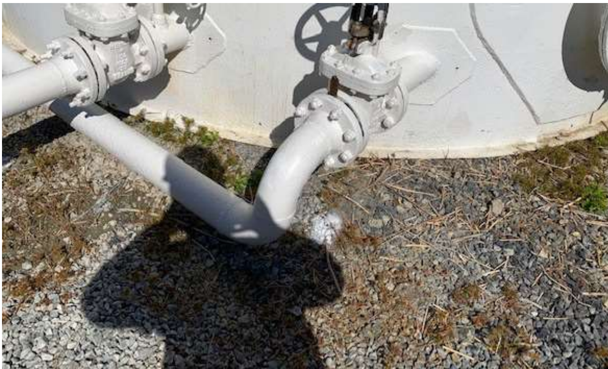
Photo 2: Photograph of flange where tank inspector identified oily residue on exterior of piping in March 2022. No clear staining observed on ground surface and no remaining residue on piping.
