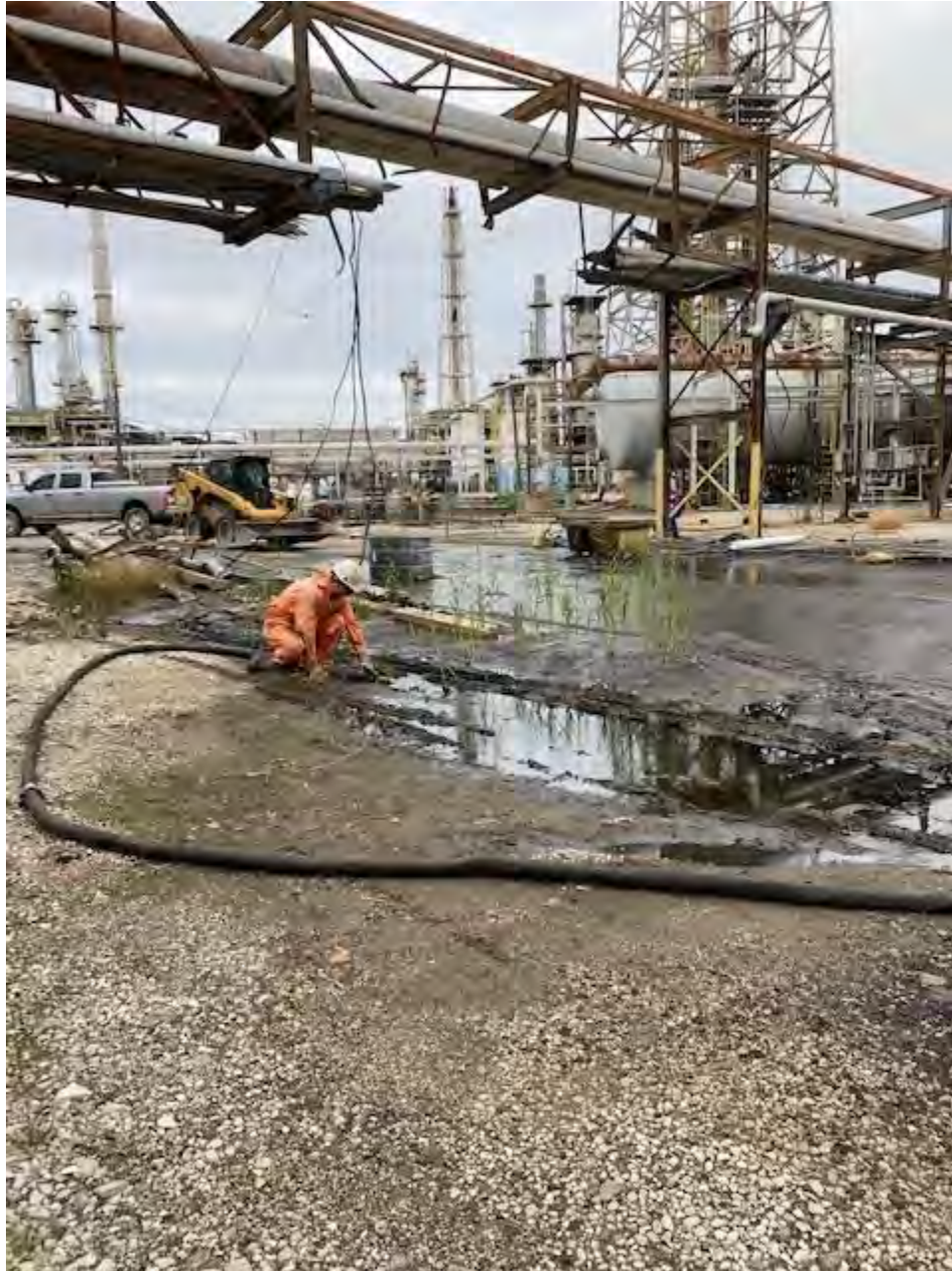
Vacuuming oil and wash water from Area 2 of the spill calculation Sheet. Water was decanted from the vacuum truck (estimated 500 gallons) and remaining oil placed in tank 272 slop oil tank for future sale.
