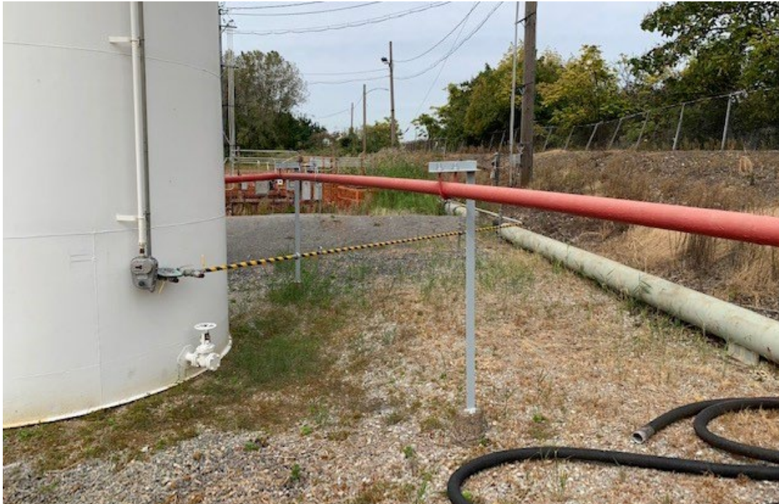
Photo 3 (September 2022): North side of Tank 056A; no staining observed.
