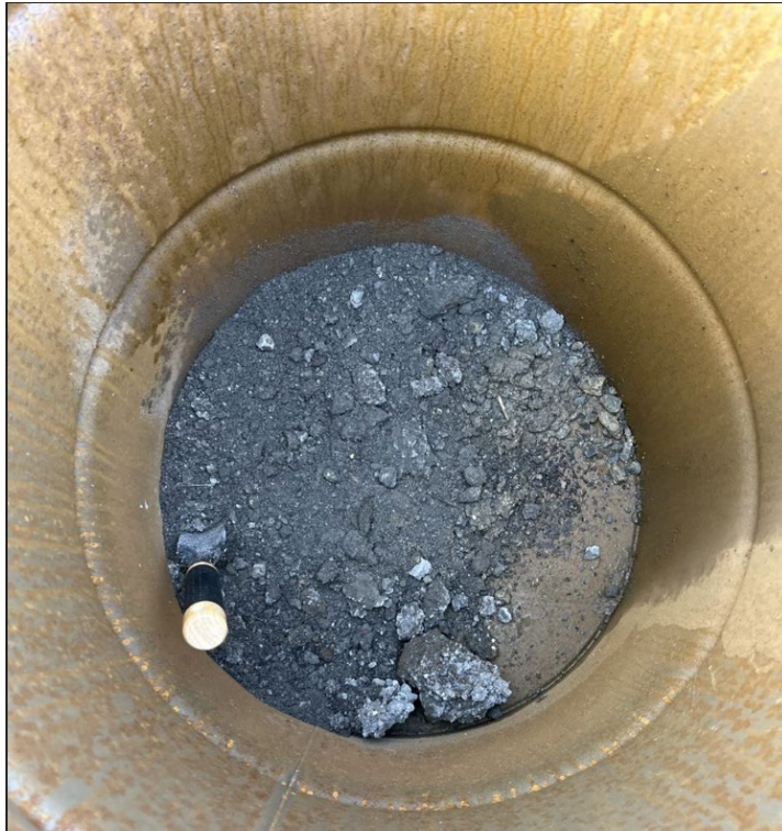
Photo 6 (February 2023): Approximately 0.5 cubic foot of soil removed from the berm beneath the valve. Material removed consists of mainly gravel with some medium sand.
