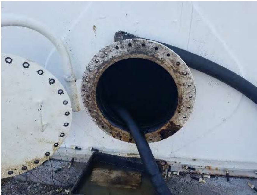
Photograph 2: View of Tank 004A (GP R 284) being cleaned.
