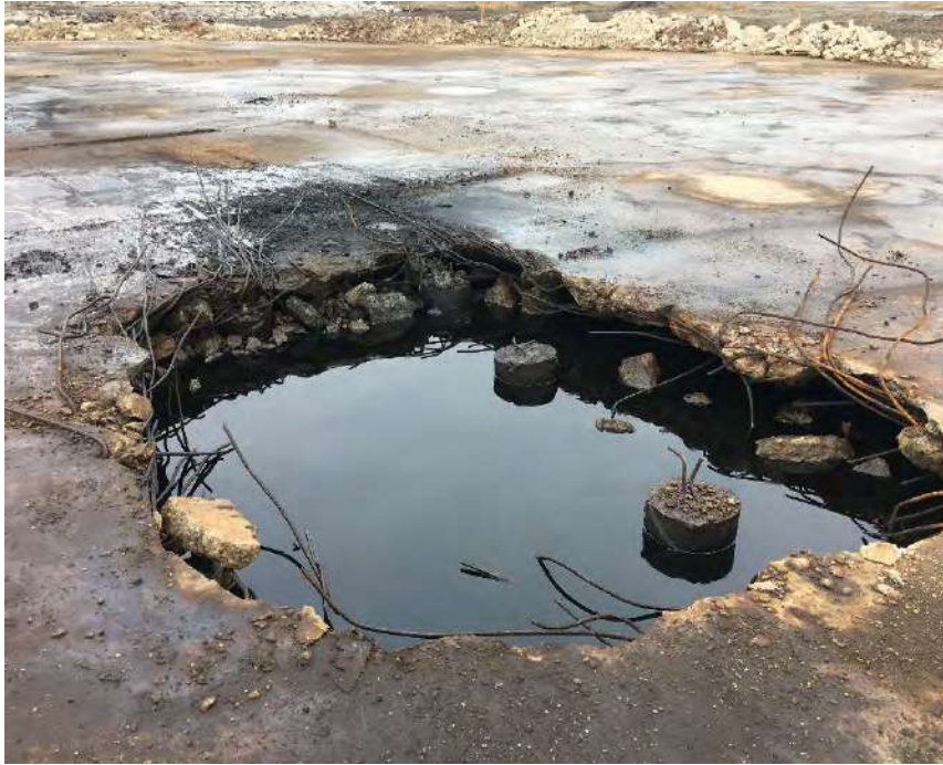
Photograph 3: View of NAPL beneath the tank foundation at Tank 025A (GP R 281).
