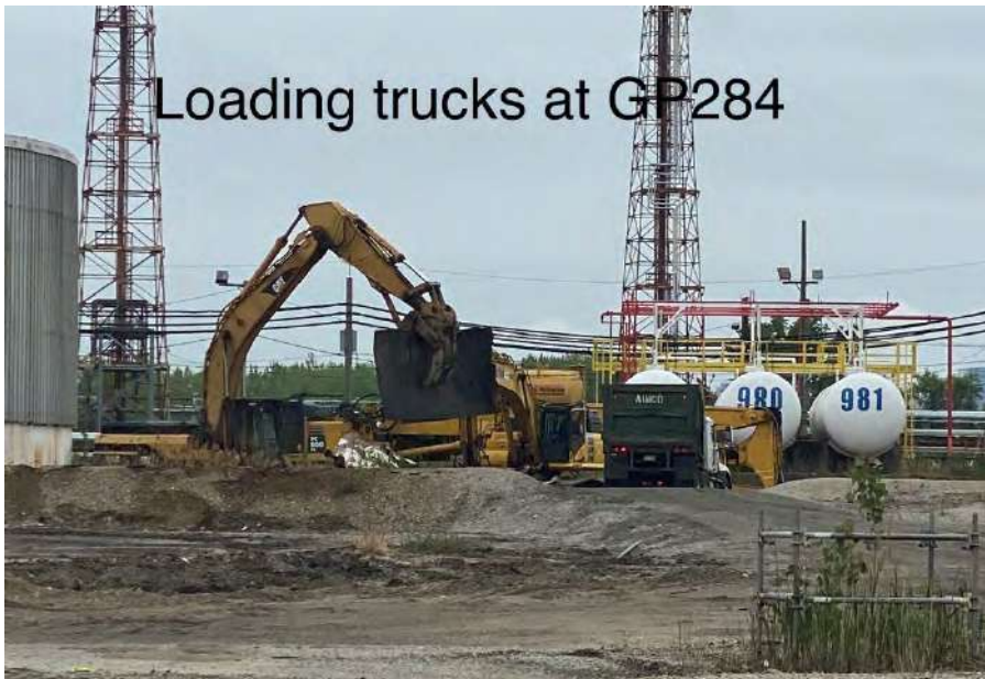
Photograph 4: View of scrap cleanup at Tank 004A (GP R 284).
