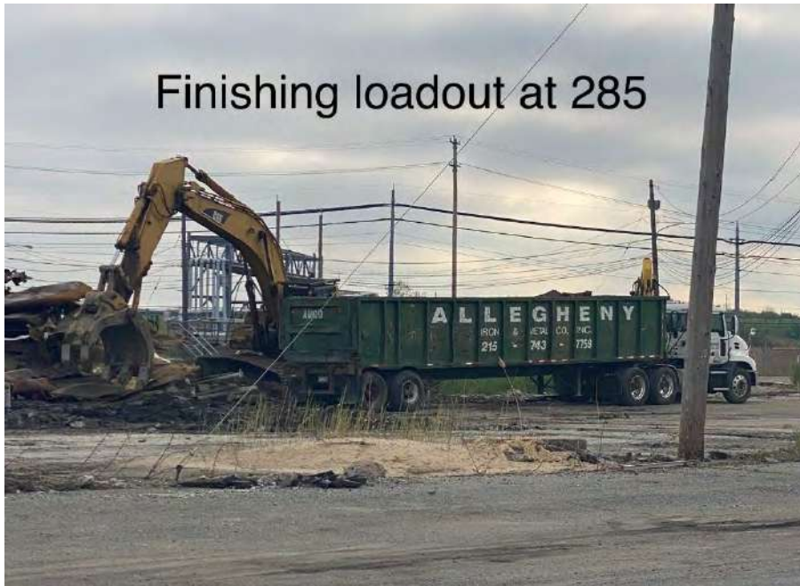
Photograph 4: View of scrap material load out at Tank 027A (GP R 285).
