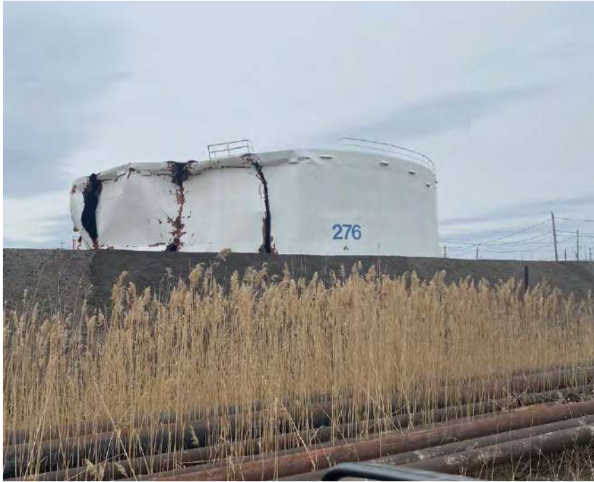
Photograph 1: View of Tank 023A (GP R 276) during demolition.
