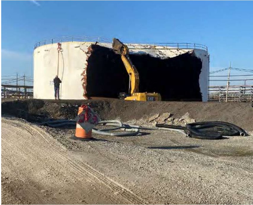
Photograph 1: View of Tank 021A (GP R 270) during demolition.
