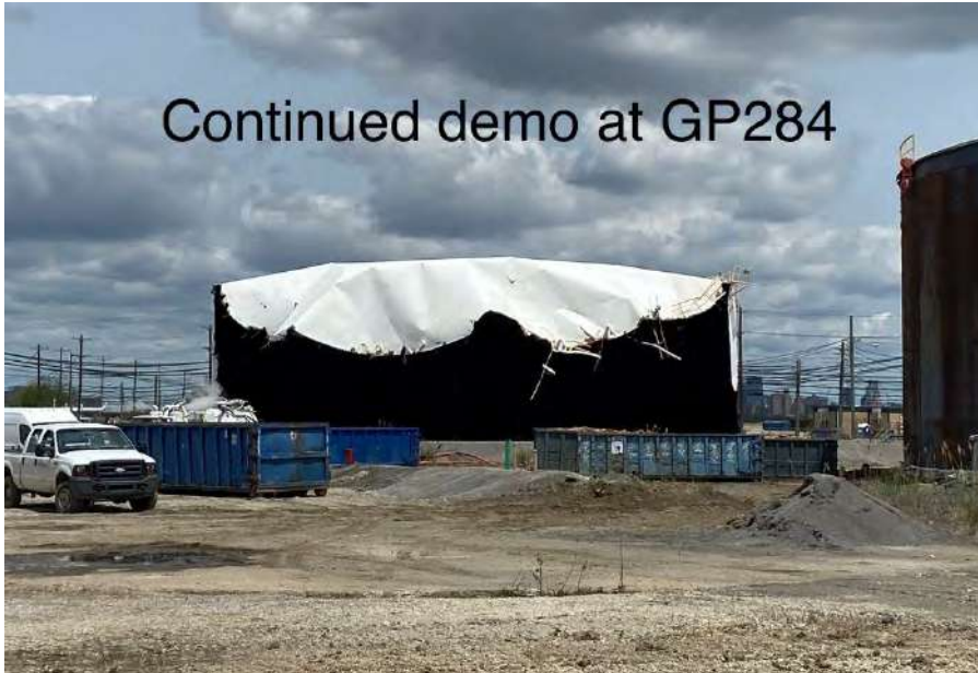
Photograph 3: View of Tank 004A (GP R 284) during demolition.
