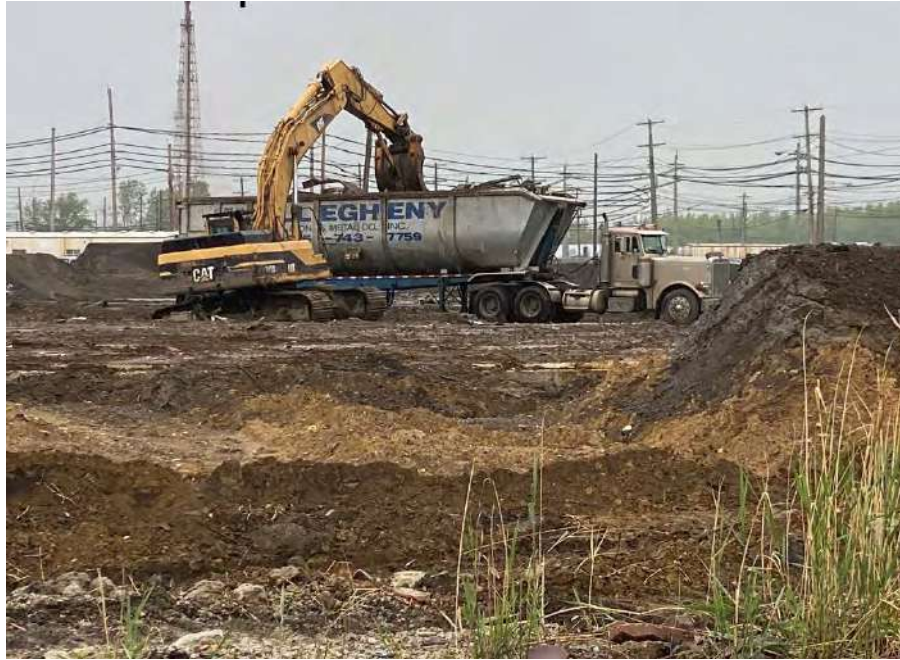
Photograph 3: View of scrap material load out at Tank 027A (GP R 285).
