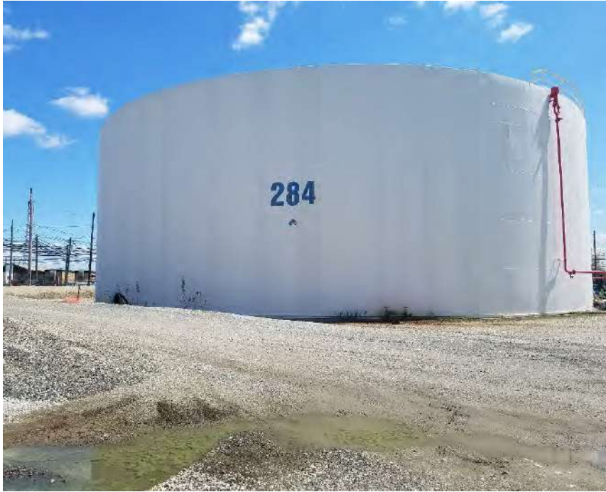
Photograph 1: View of Tank 004A (GP R 284) prior to demolition.
