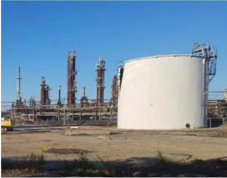
Photograph 1: View of Tank 005A (GP R 1117) during demolition.
