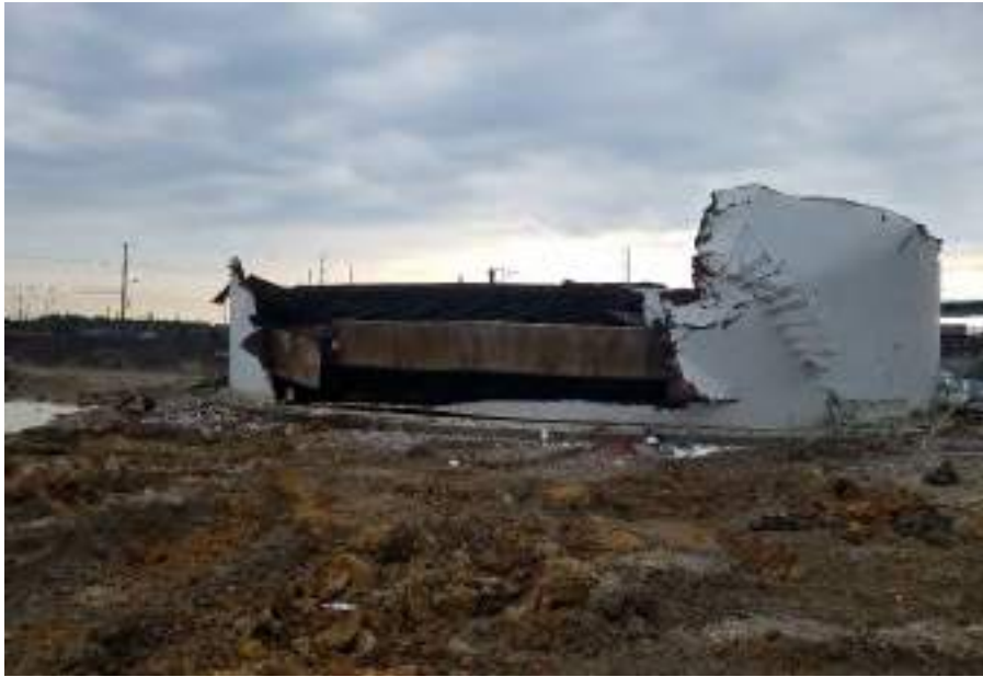
Photograph 3: View of Tank 005A (GP R 1117) during demolition.
