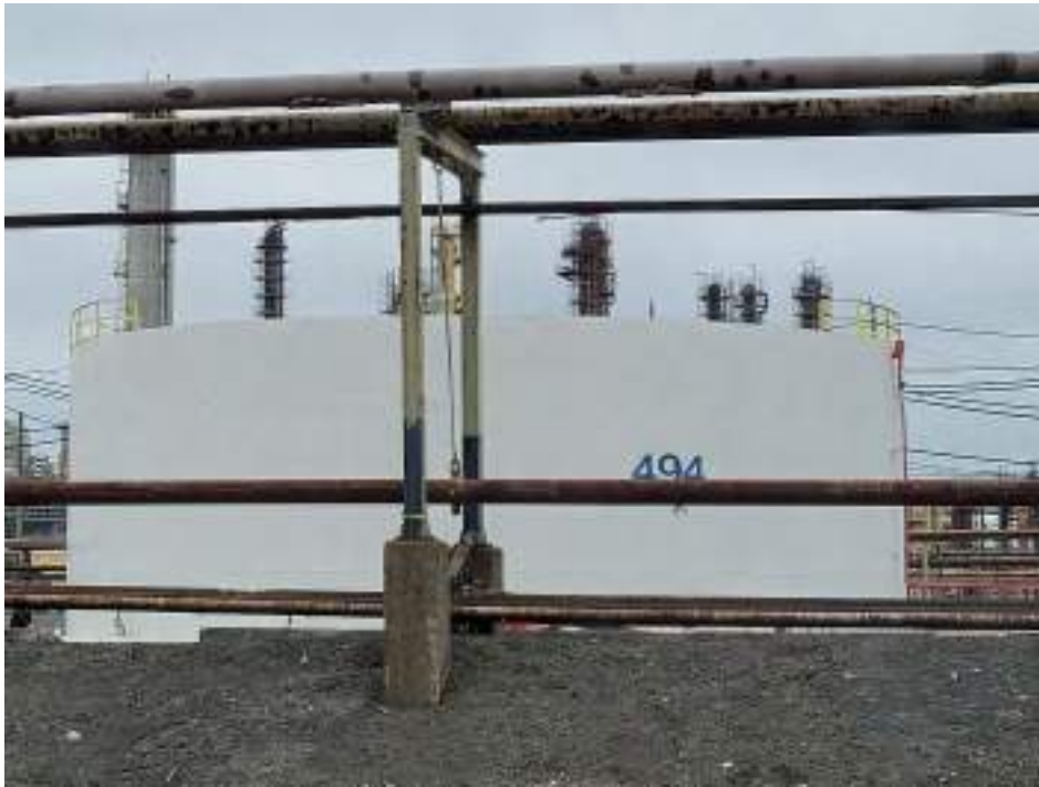
Photograph 1: View of Tank 029A (GP R 494) prior to demolition.
