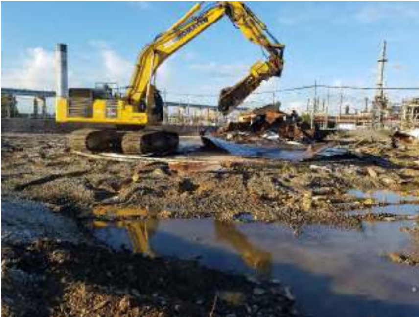
Photograph 2: View of scrap piles and the concrete pad during demolition.
