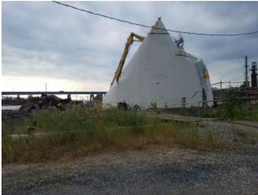
Photograph 2: View of Tank 005A (GP R 1117) during demolition.
