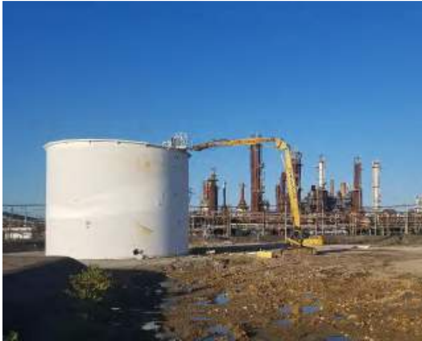
Photograph 1: View of Tank 030A (GP R 1116) during demolition.
