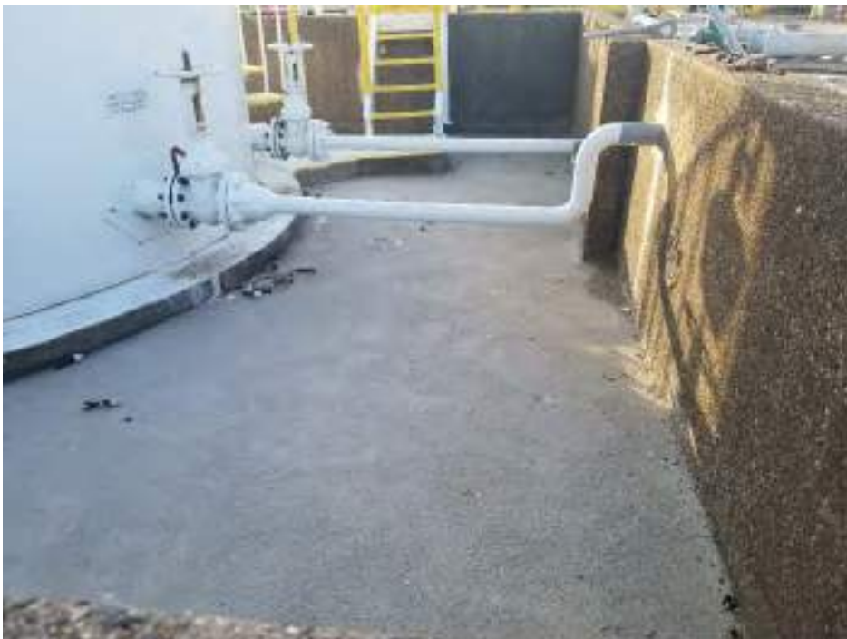
Photograph 2: View of Tank 033A (GP R 1088) piping prior to demolition.
