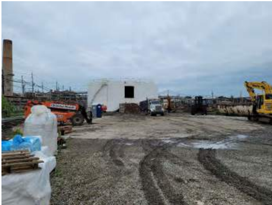
Photograph 2: View of Tank 029A (GP R 494) during demolition.
