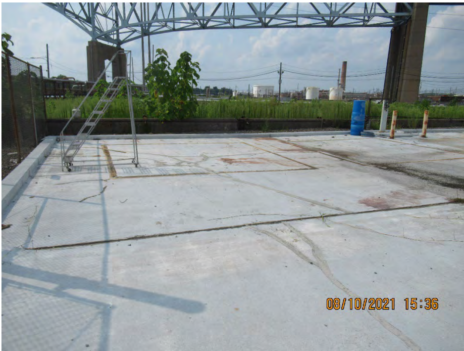
Photograph 2: View of Girard Point Hazardous Waste Storage Pad with notable staining prior to paving.
