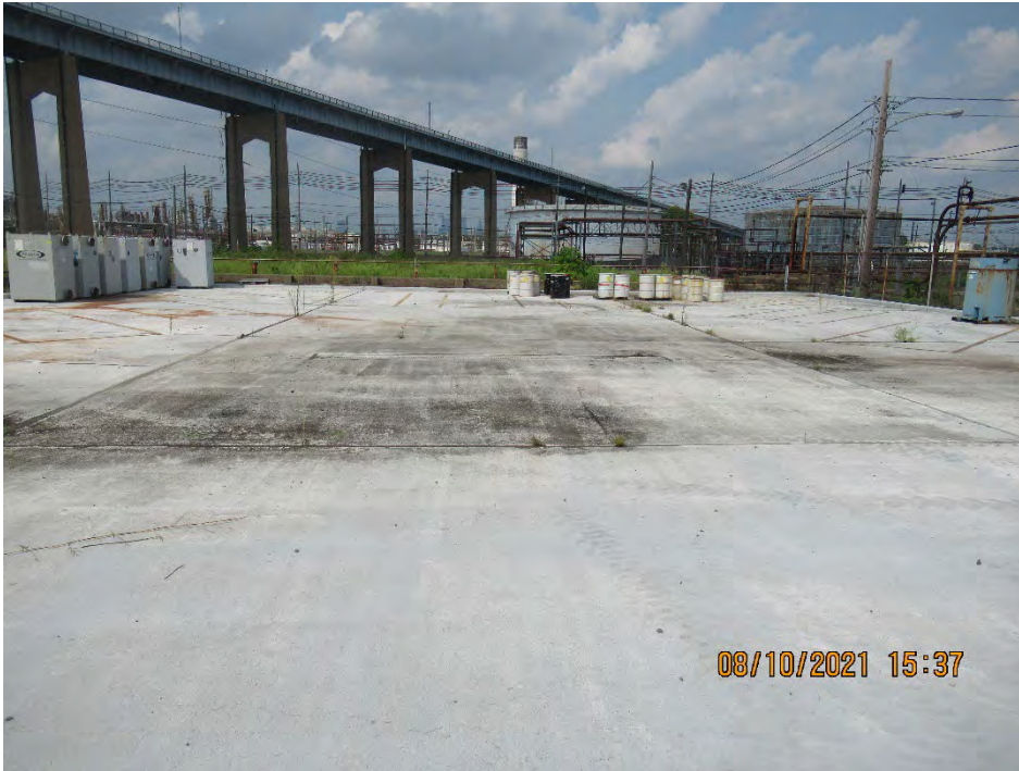
Photograph 1: View of Girard Point Hazardous Waste Storage Pad with notable staining prior to paving.
