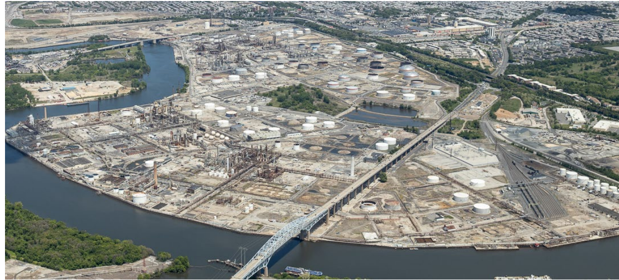
Entire Refinery, May 2021
