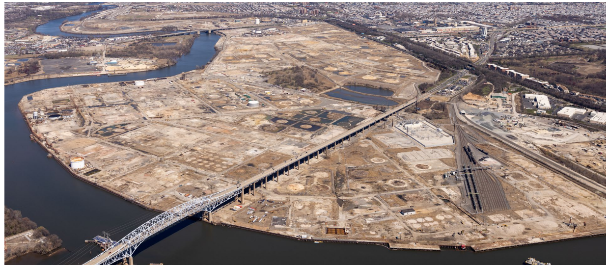
Entire Refinery, March 2023
