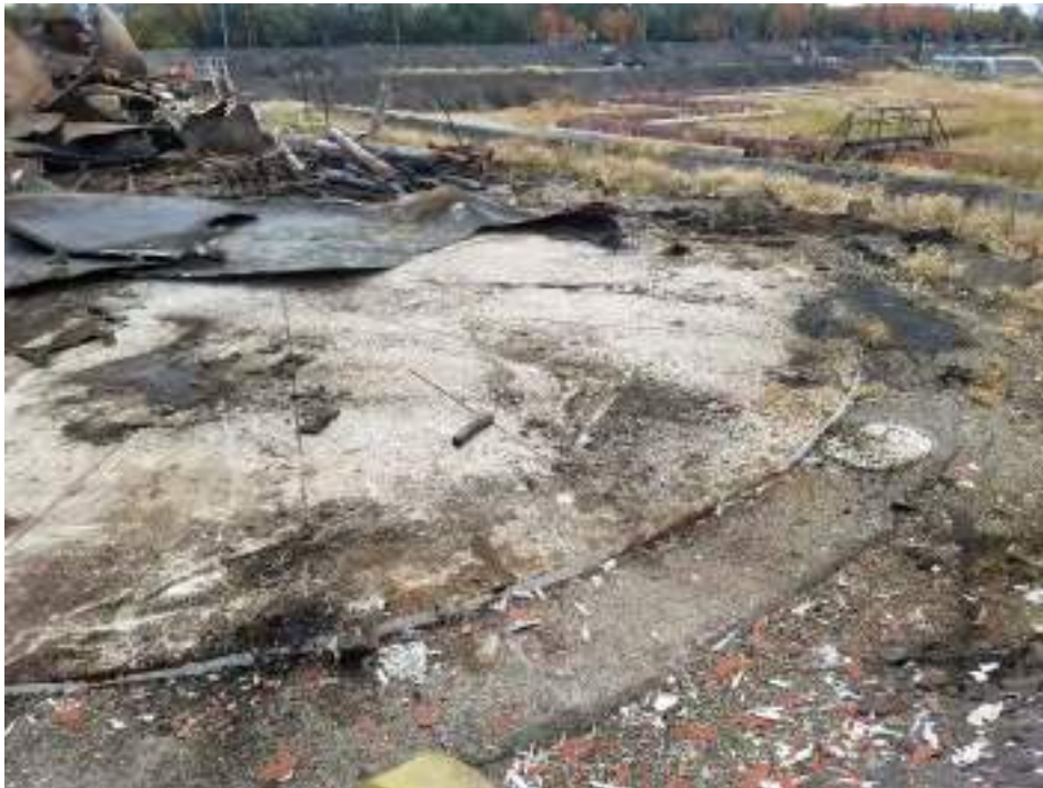
Photograph 3: View of scrap piles and Tank 040A (PB 191) following demolition.
