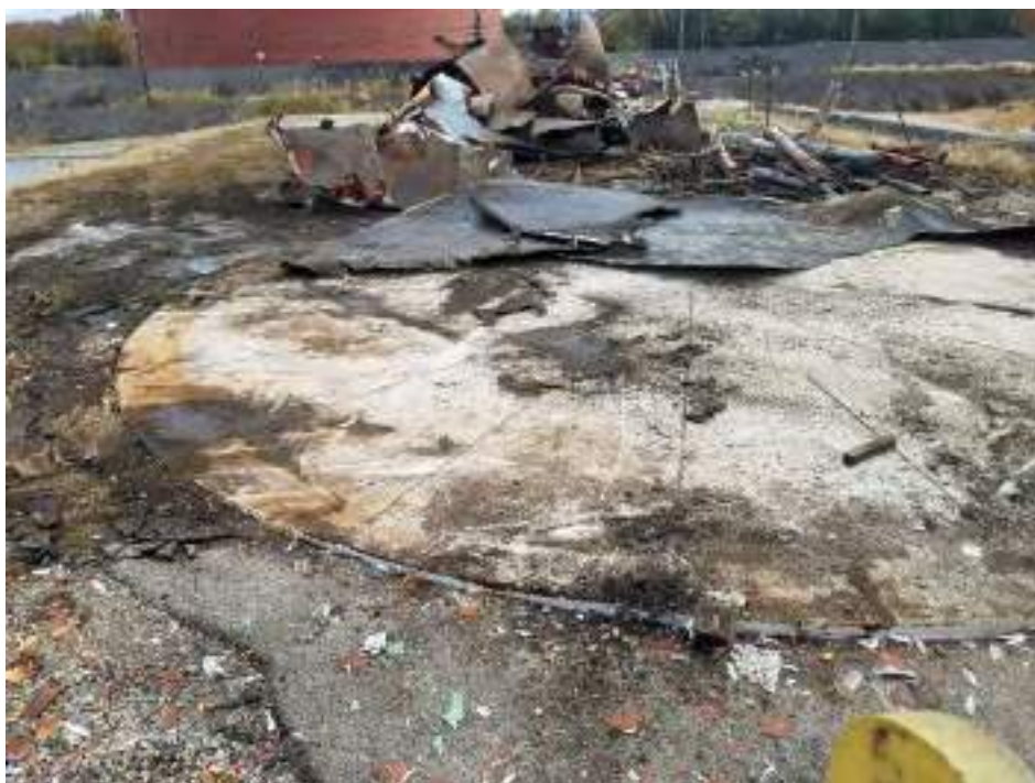
Photograph 2: View of scrap piles and Tank 040A (PB 191) following demolition.
