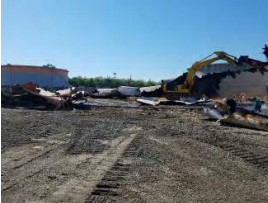
Photograph 5: View of scrap piles during demolition.
