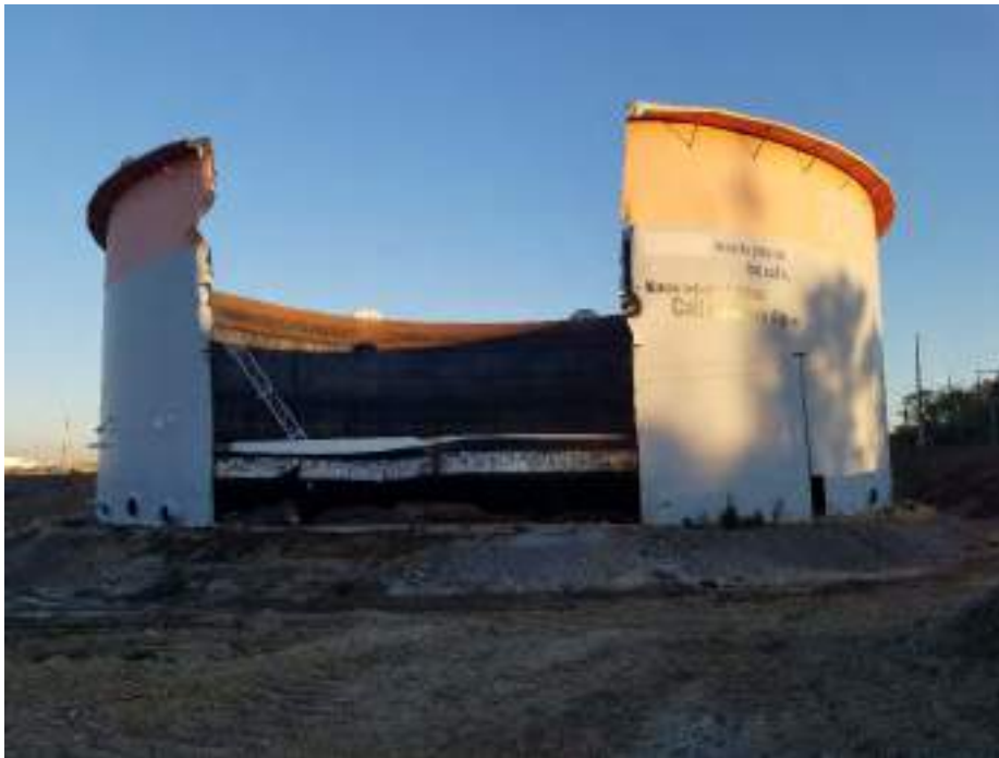
Photograph 2: View of Tank 057A (PB 883) during demolition.
