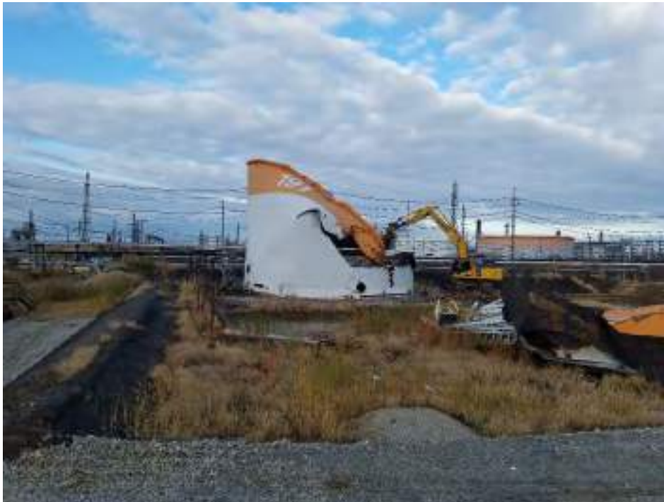
Photograph 1: View of Tank 040A (PB 191) during demolition.
