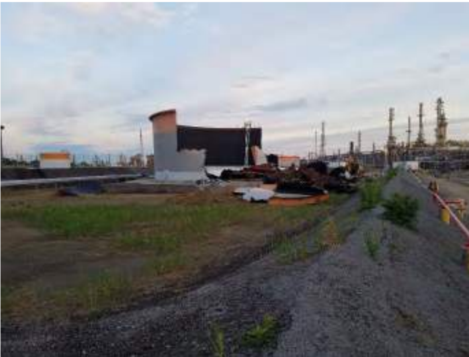
Photograph 2: View of Tank 056A (PB 882) during demolition.
