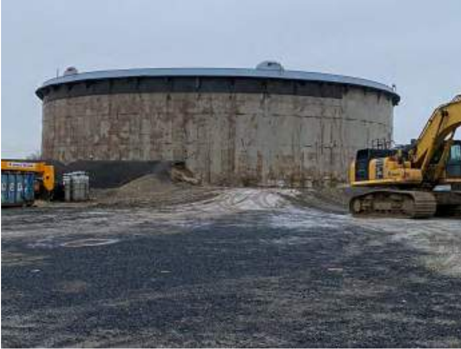
Photograph 1: View of Tank 086A (PB 843) during demolition.
