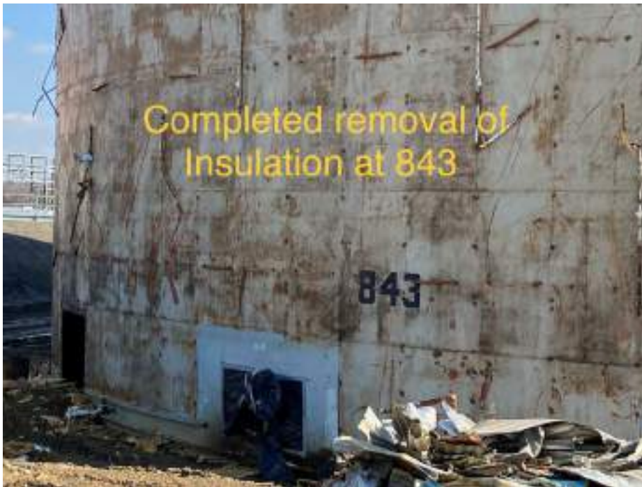
Photograph 2: View of Tank 086A (PB 843) during demolition.
