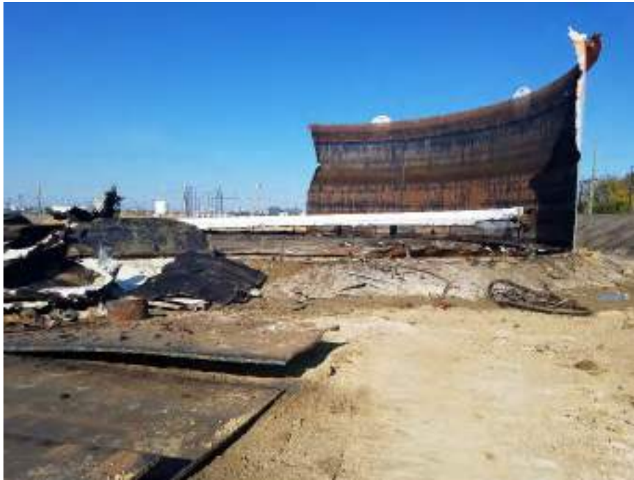
Photograph 3: View of Tank 057A (PB 883) during demolition.
