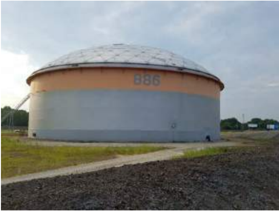
Photograph 1: View of Tank 012A (PB 886) prior to demolition.
