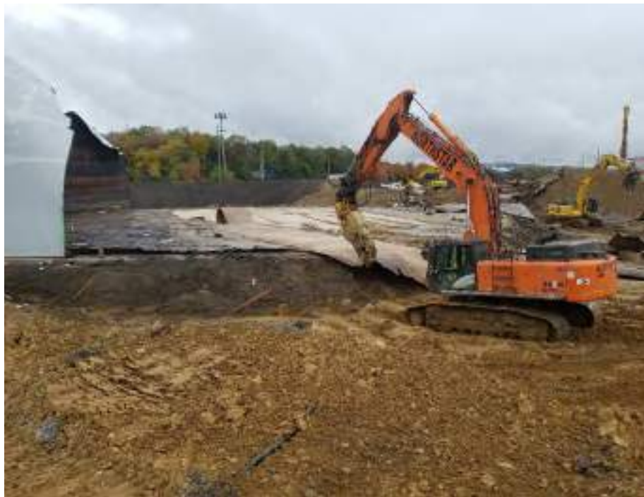
Photograph 4: View of Tank 057A (PB 883) during demolition.
