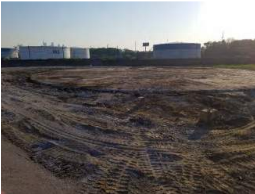
Photograph 6: View of the concrete pad following demolition.
