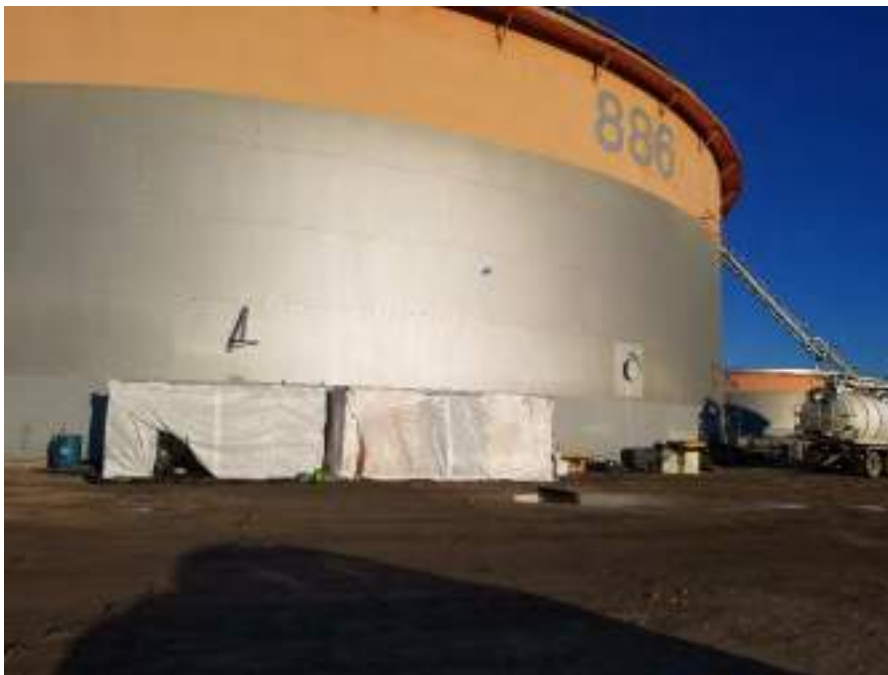
Photograph 2: View of Tank 012A (PB 886) prior to demolition.
