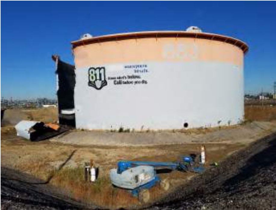
Photograph 1: View of Tank 057A (PB 883) during demolition.
