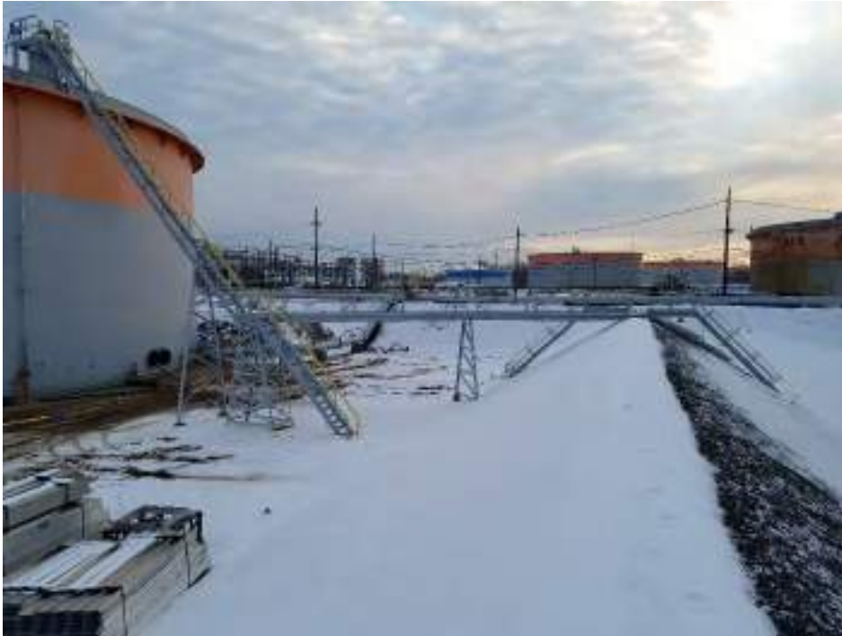
Photograph 3: View of piping for Tank 054A (PB 841) prior to demolition.
