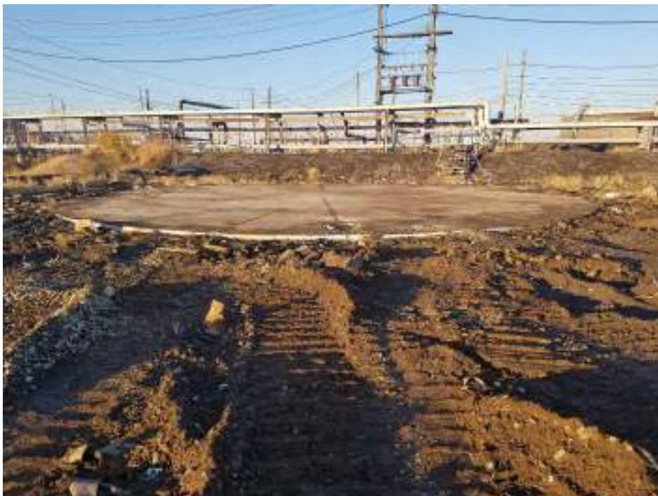
Photograph 4: View of the concrete pad following demolition.
