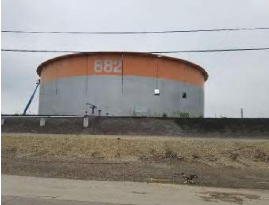
Photograph 1: View of Tank 056A (PB 882) prior to demolition.
