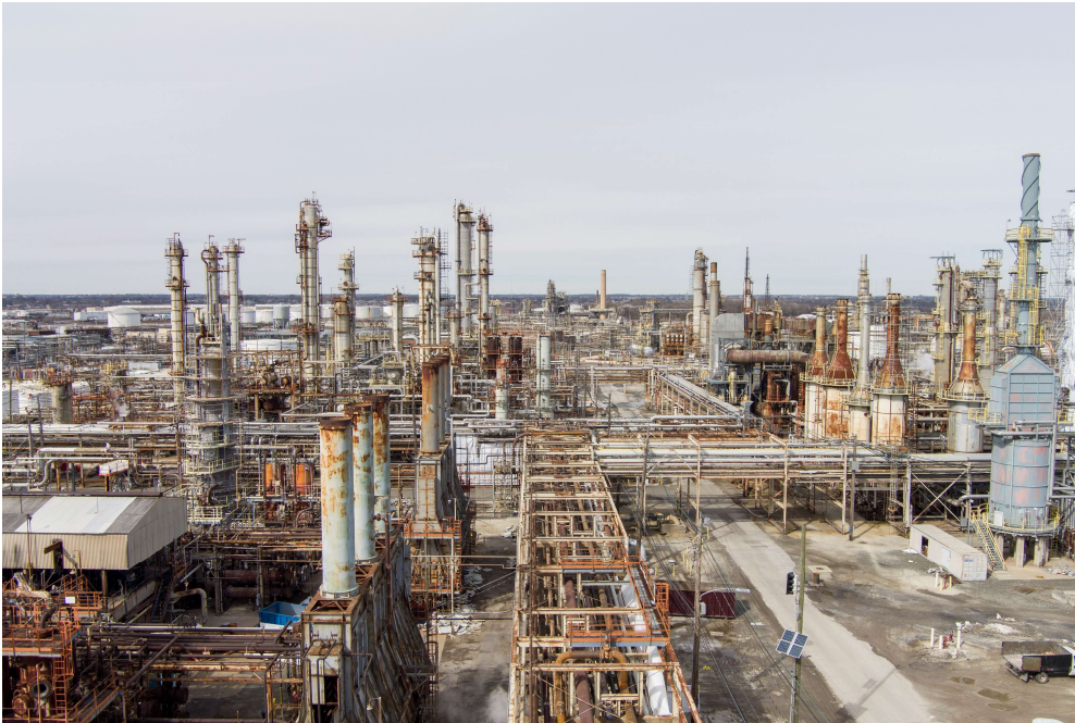
Distillate Processing Unit before demolition
