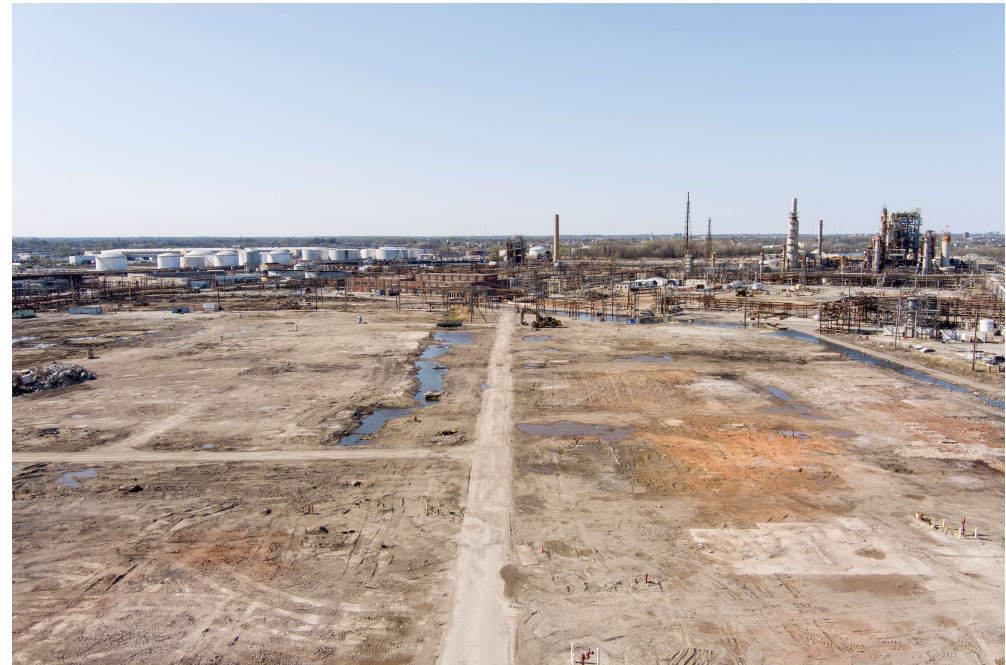
Distillate Processing Unit after demolition
