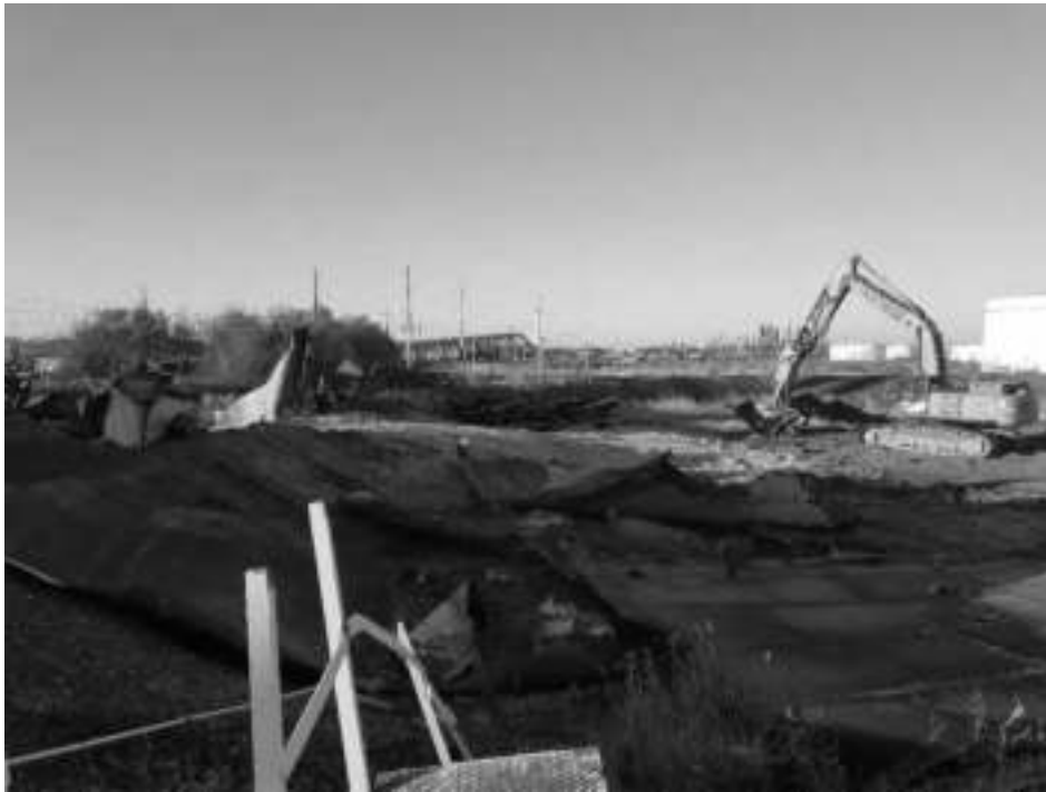
Photograph 3: View of scrap pile.
