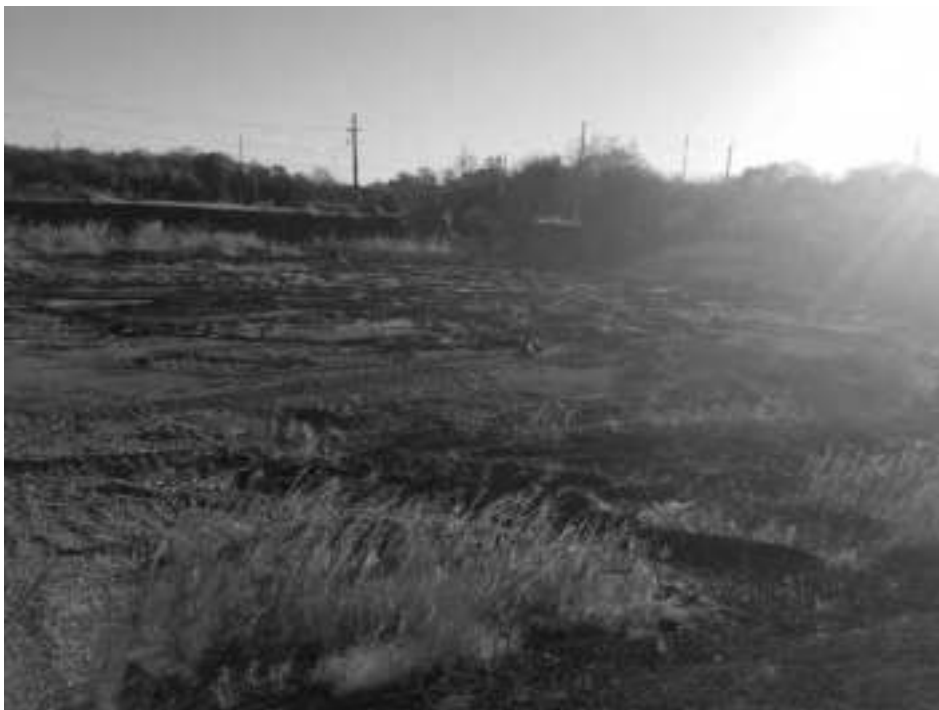
Photograph 4: View of soil following demolition.
